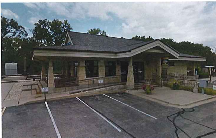
Village of Palos Park Metra Station
