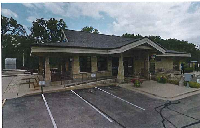
Village of Palos Park Metra Station
