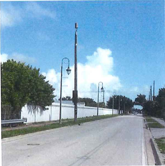
Wood Utility Pole Installation
