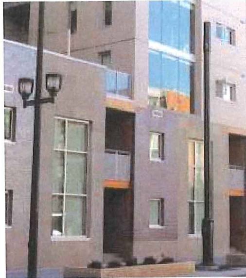
New Utility Pole with Stealth Concealment
