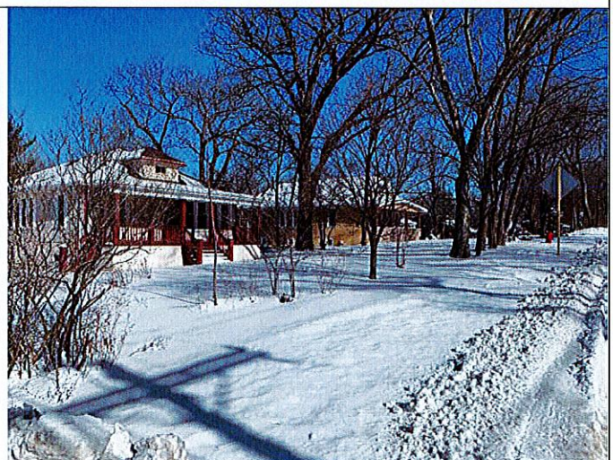
View of Site at 123rd
