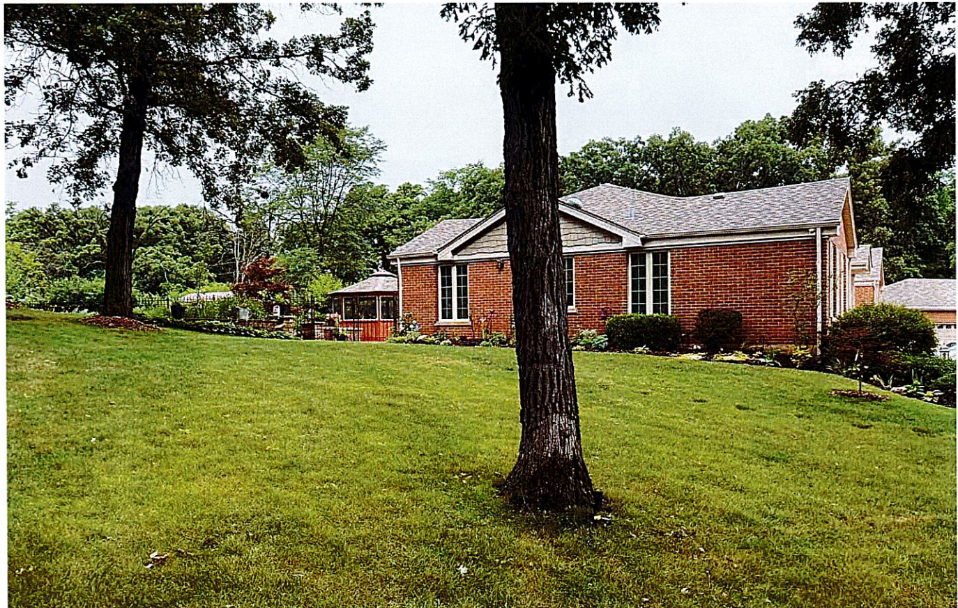
South end of property, facing north
