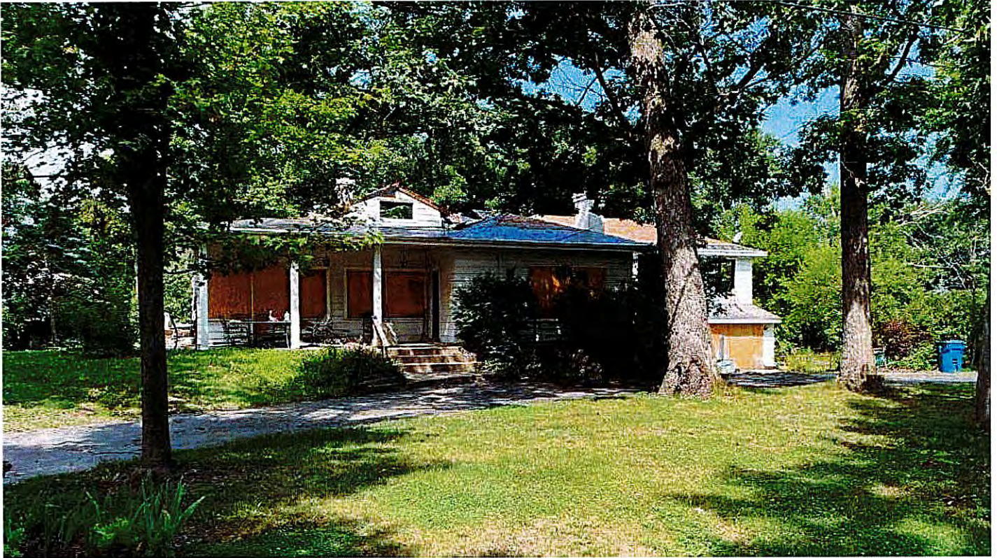
Front elevation of home
