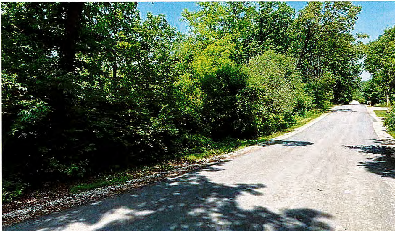
91 st Avenue, north of intersection with 126 th , facing north-northwest
