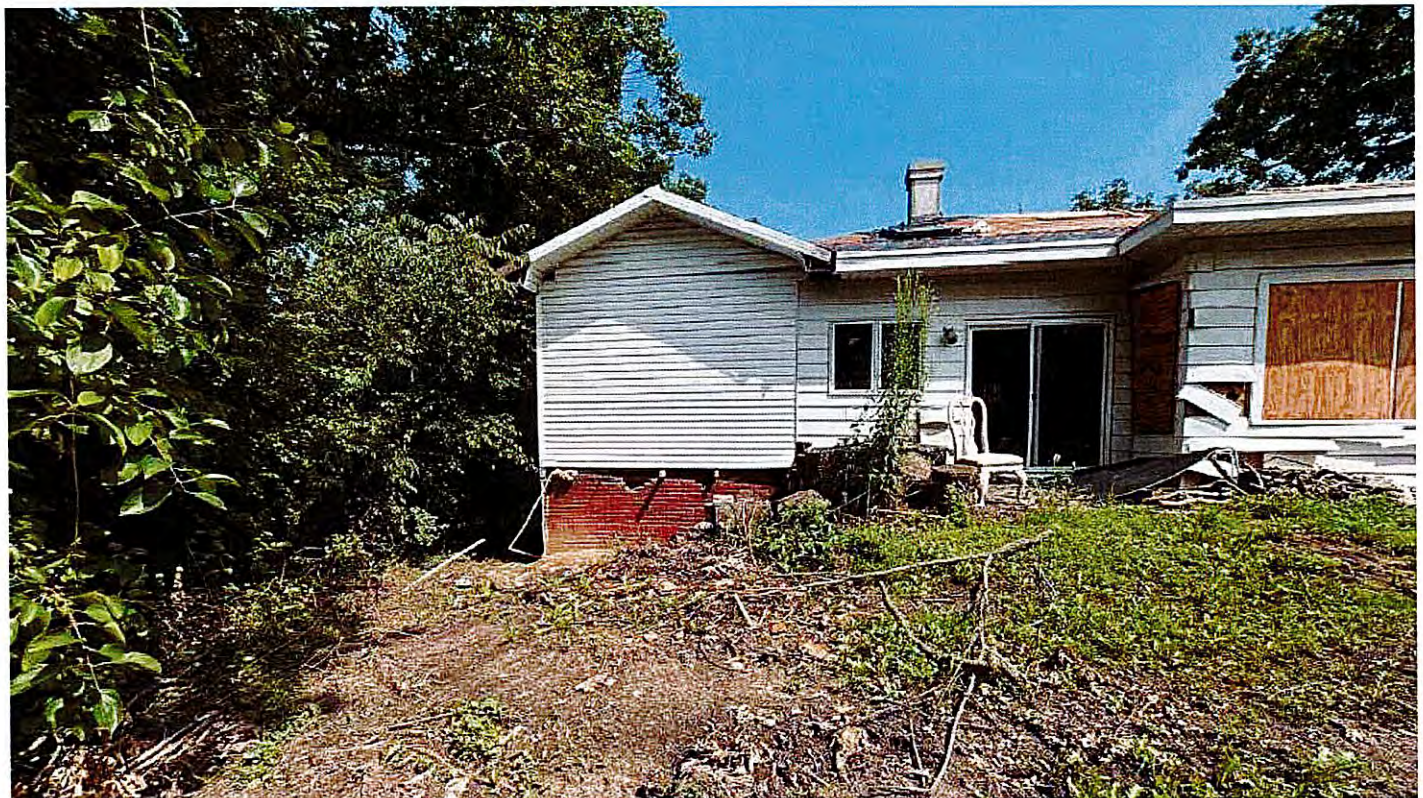
South elevation of the home, along rear property line; facing north
