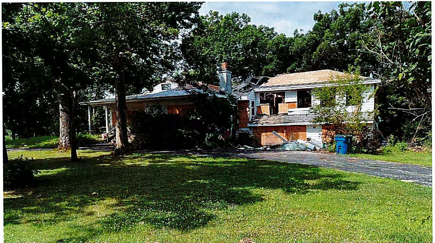
Front elevation of home
