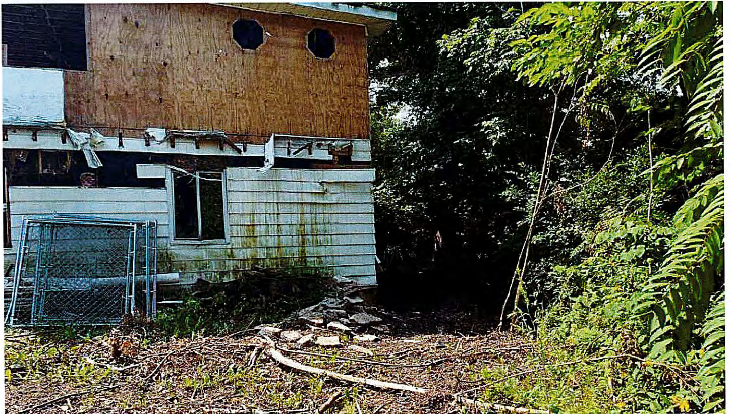
North elevation of the home, along rear property line; facing south
